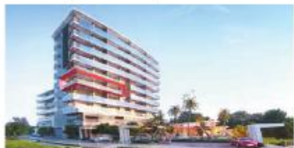
East Quays Four Harbour Quays, Gold Coast. Completed 2016 Value $29m
