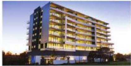
Zephyr at Harbour Quays Harbour Quays, Gold Coast. Completed 2014 Value $33m
