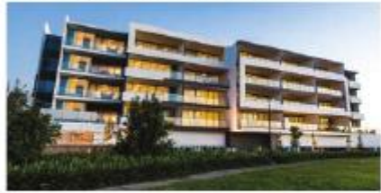
Sirocco at Harbour Quays Harbour Quays, Gold Coast. Completed 2013 Value $18m
